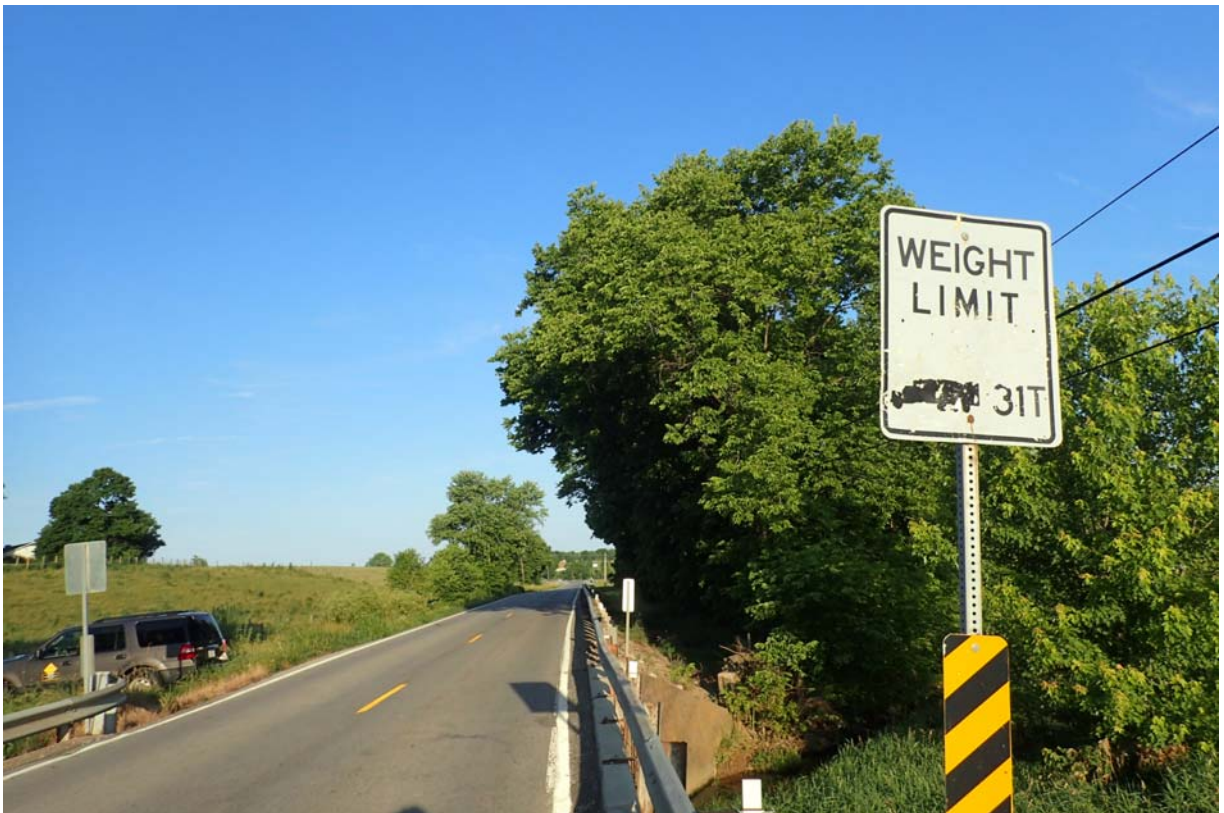
View of the weight limit posting near abutment 2.
