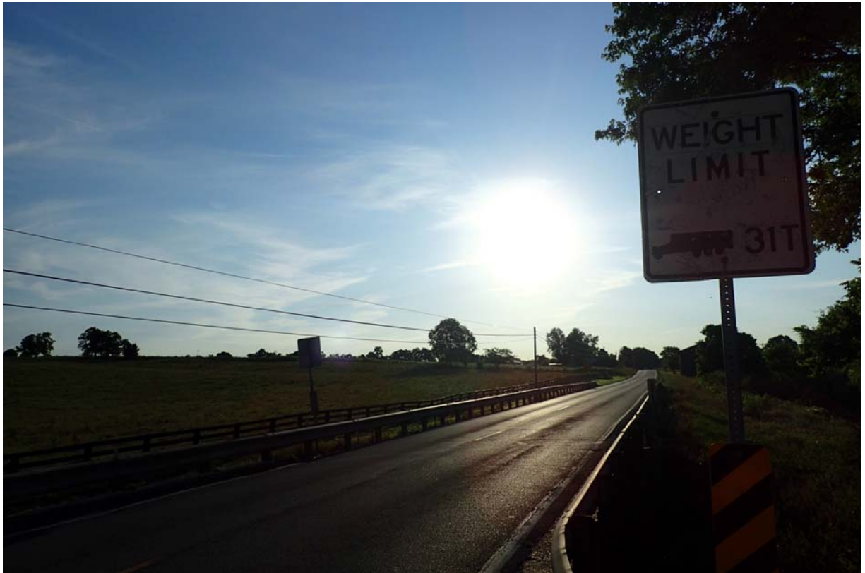
View of the posting sign near abutment 1.
