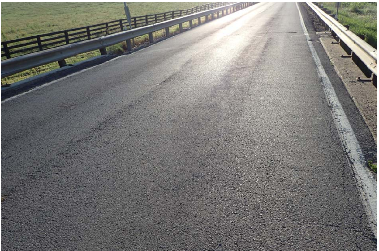
Typical view of the asphalt wearing surface.
